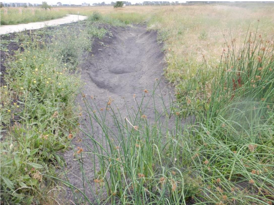
Photo 6: Erosion on the margin of the creek corridor within 165-195 O'Herns Road.
