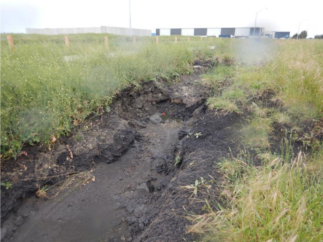
Photo 5: Erosion on the margin of the creek corridor within 165-195 O'Herns Road.
